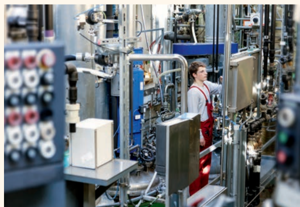
Fig. 3: Employees at the chemical synthesis plant of 3M in Seefeld.
