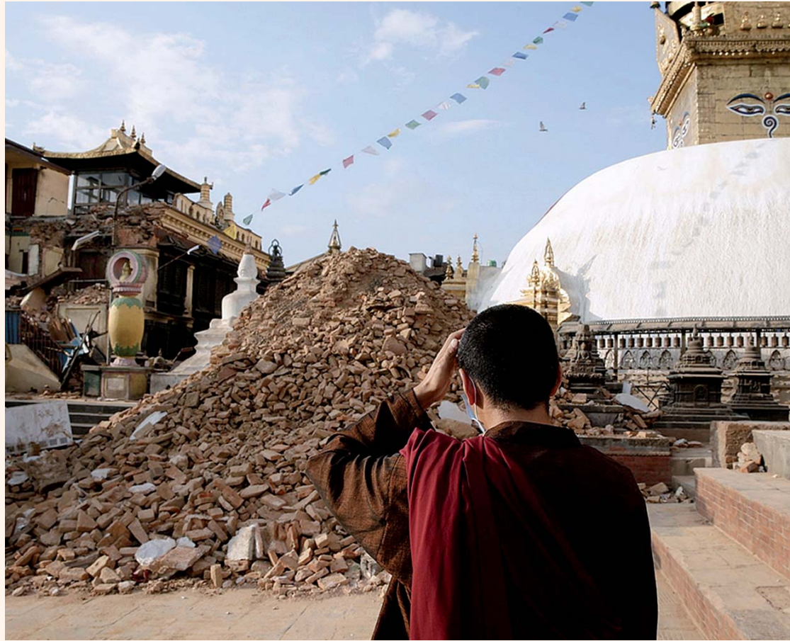
Monk looking at destruction caused by the 25 April earthquake in the Nepalese capital Kathmandu. Damages are estimated at US$200 million. © Narendra Shrestha/EPA
