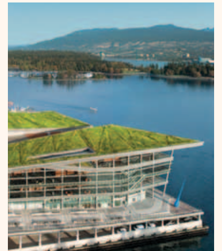
The Vancouver Convention Centre, its 'green' roof clearly visible, is host site of the 2016 Pacific Dental Conference. Photo/Provided by the Vancouver Convention Centre
