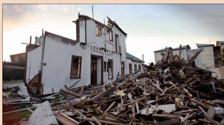
Earthquake-damaged buildings in Christchurch, New Zealand. The devastations caused by the disaster in 2011 also had an effect on the dental infrastructure. NZDA's Donna Batchelor explains. (DTI/Photo Alexandralaw1977) ▶ ASIA NEWS, page 2
