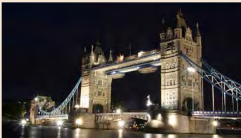
London's iconic Tower Bridge
